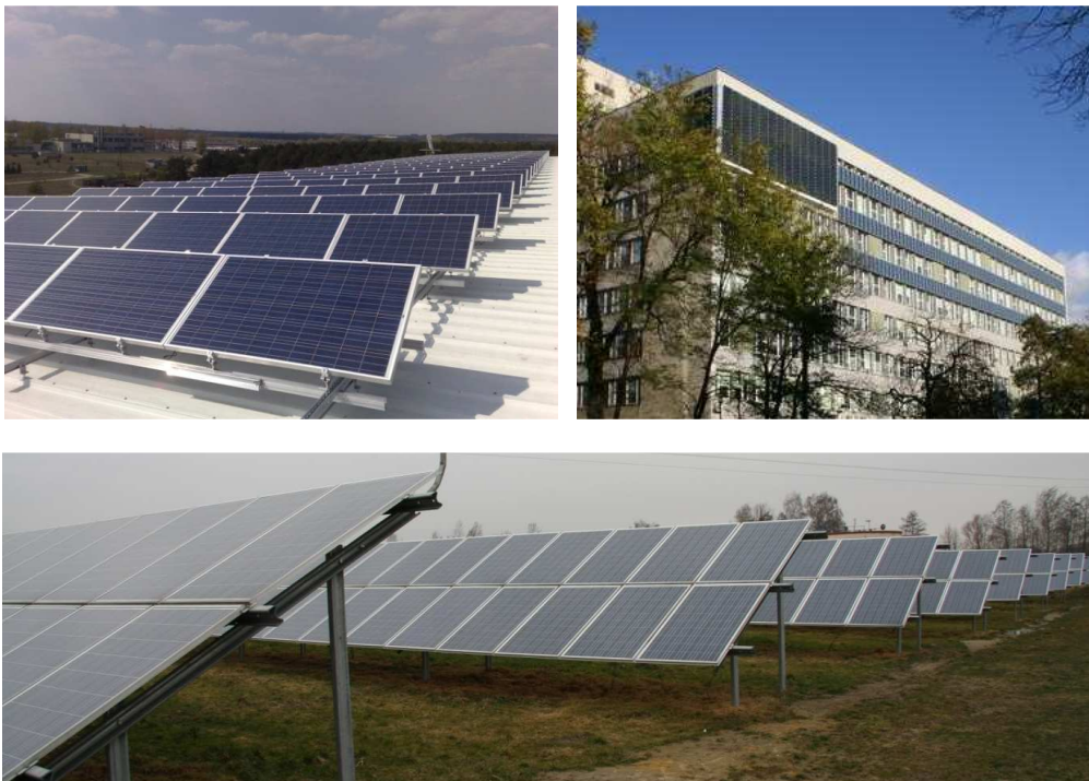
Fig. 44. 80,5 kW p PV system used by the FROSTA company in Bydgoszcz. (left). Faculty of Environmental Engineering of the Warsaw University of Technology - facade of the building (right). 1 MWp, grid connected PV system located in Wierchosławice community (bottom)
